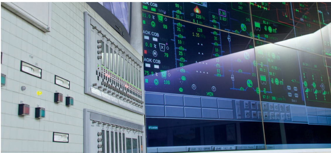
A modern power station control room.
